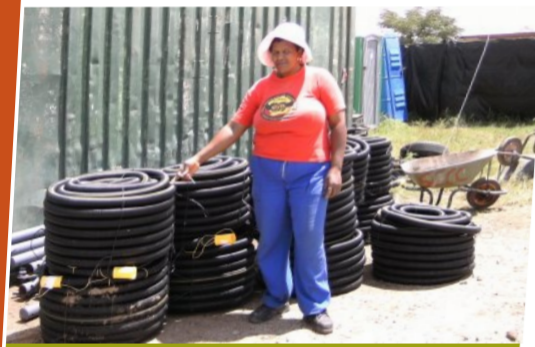
Bringing street lighting to Evaton
